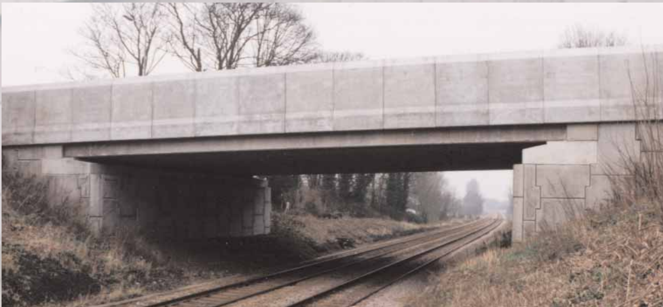
Harford Rail Bridge, Norwich. UK.
