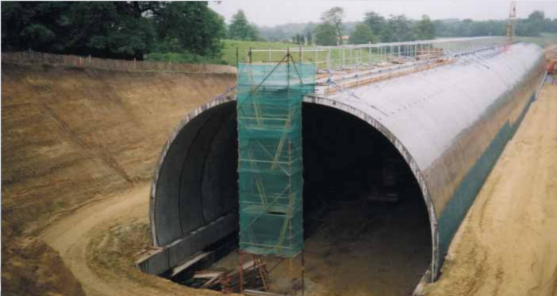
Contract 420, Channel Tunnel Rail Link, Kent. UK.
