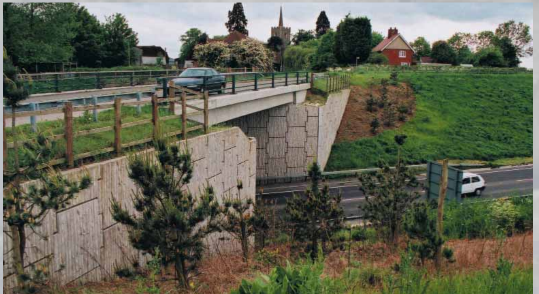
Church Lane Overbridge, Bishop's Stortford. UK.
