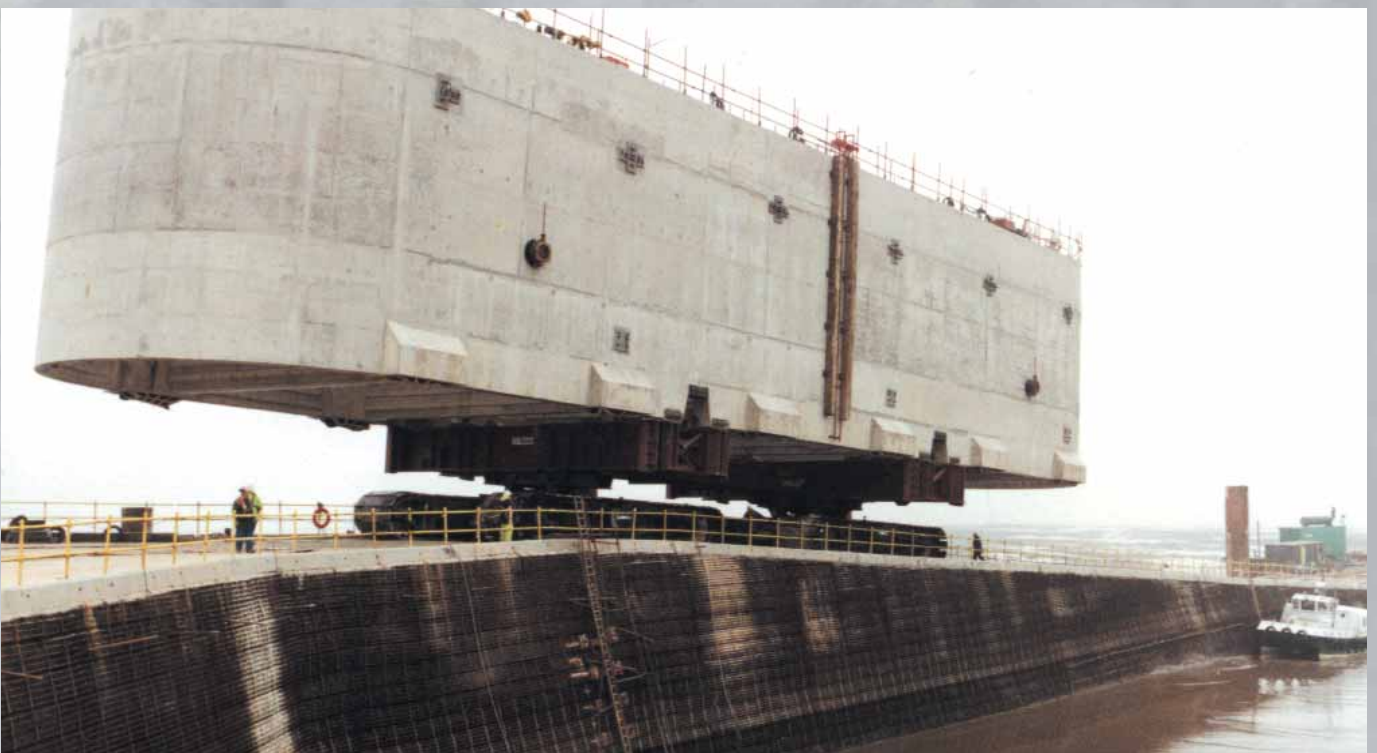
Ro-Ro Ramp, Second Severn Crossing. UK. High Commendation: British Construction Industry Awards 1993.
