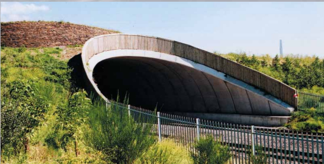
Millennium Coastal Park Land Bridges, Llanelli. UK. Winner: 1998 George Gibby Award by the Institute of Civil Engineers South Wales Association. Shortlisted: 1999 British Construction Industry Awards
